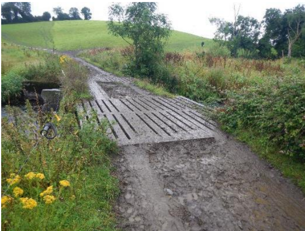
Photo 55. A track crossing and slatted farm bridge creates a small pollution issue but as the track is pretty much disconnected from the bridge, the issue is limited (53.986492, - 6.554433). Small cross drains could be cut into (or raised across) the track on LB side to ensure that surface runoff from the hill drains to rough ground, not the watercourse.
