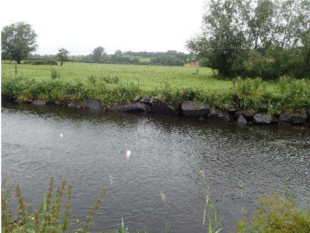
Photo 85. A short distance downstream there was evidence of more substantial bank protection work using large pitched rocks for rip-rap adjacent to the LB. This would appear an excessive measure to reduce bank erosion when a simple stock fence and narrow buffer zone would have provided adequate protection - also cover and food for fish and invertebrates. Although it could be argued that pitched stone provides gaps and micro niches for small fish, it is a poor substitute for a naturally functioning "soft" margin and invariably leads to further erosion problems elsewhere.
