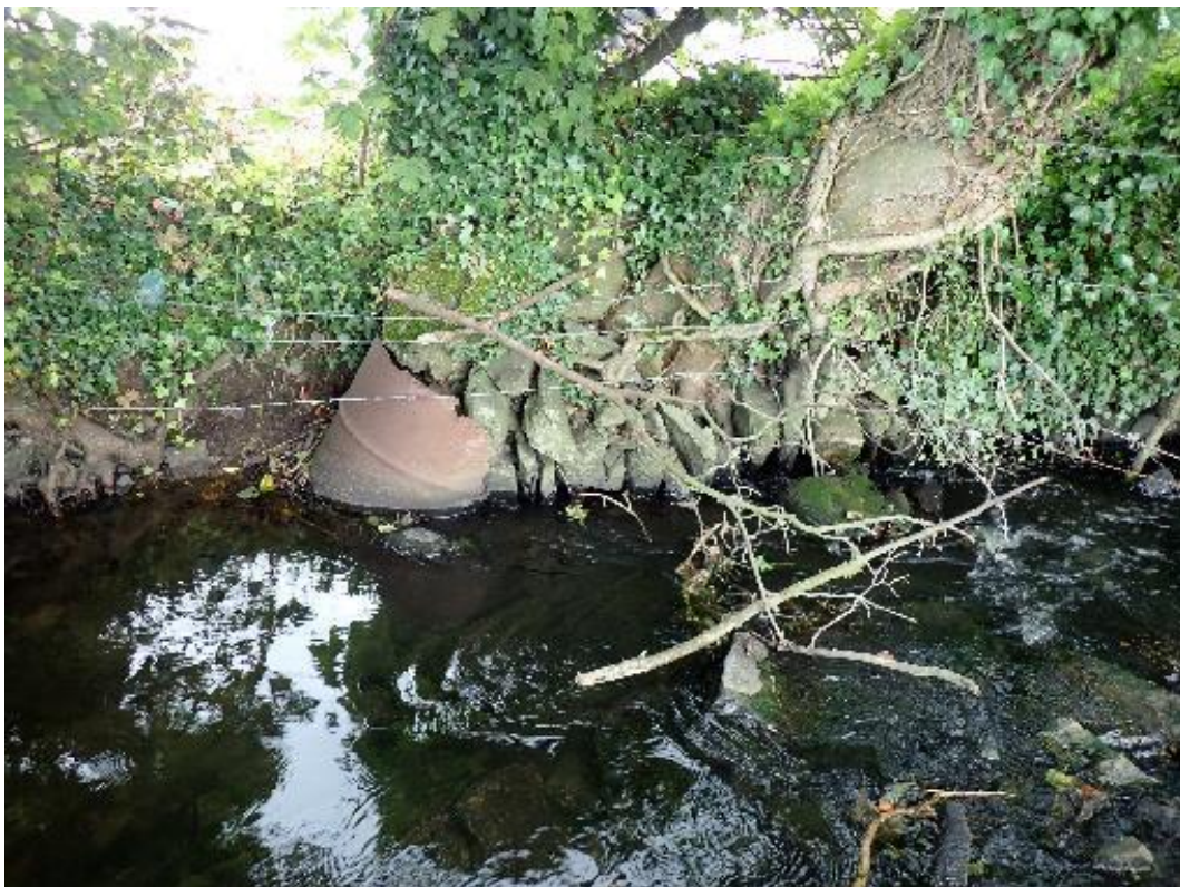
Photo 130. A section of the lower Ballykelly with pitched stone revetment, a legacy of enthusiastic modification.
