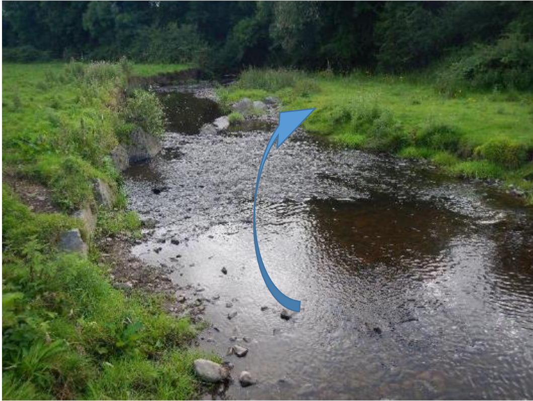
Photo 123. Around 54.139052, -6.640593, what appears to be a weir is actually the remains of failed bank protection, where the river has broken through from its previous course (blue arrow). Flow is now being directed into the bank by the failed revetment which acts as a flow deflector, which will be a particular issue at high flows. Consequently, the bank d/s is eroding at an accelerated rate.
