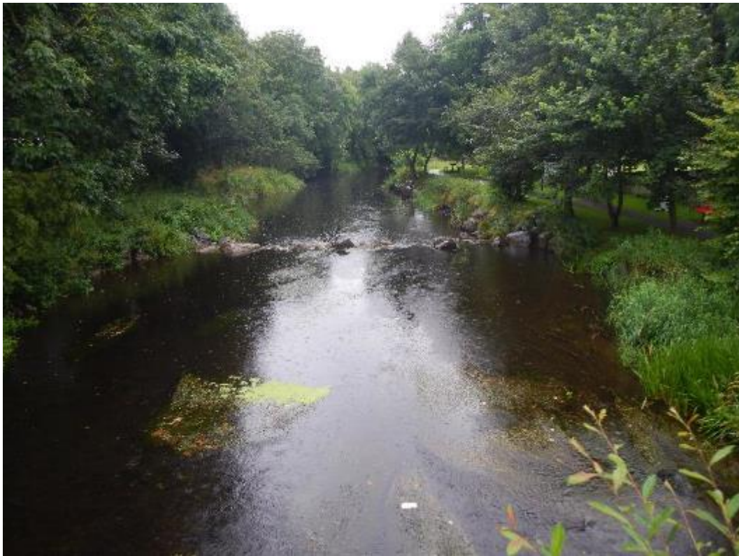
Photo 44. The larger weirs in Inniskeen not only degrade the habitat u/s and d/s, they create an impediment to the u/s and d/s migration of fish, particularly in low flows. Juvenile fish dropping down the river are often deterred by such structures, delaying their progress d/s and making them an easy target for predators.
