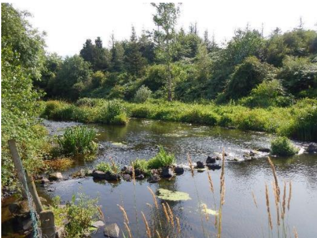
Photo 12. A weir at (54.0339750, -6.6217200) impounds flow u/s and degrades local habitat. Unlike natural pools, the additional depth created upstream of the weir is at the expense of flow diversity, leading to a reduction in habitat quality for flow-loving salmonids. Weirs also trap sediment, resulting in the reach u/s becoming much shallower over time. Ideally, this weir would be removed, or a portion notched down to bed level on the RB side, to remove the impoundment, allow free sediment transport and encourage bed scour. Prioritising flow down the RB channel d/s would encourage the reinstatement of a bend. A pasture pump or other alternative watering option is likely to be required.
