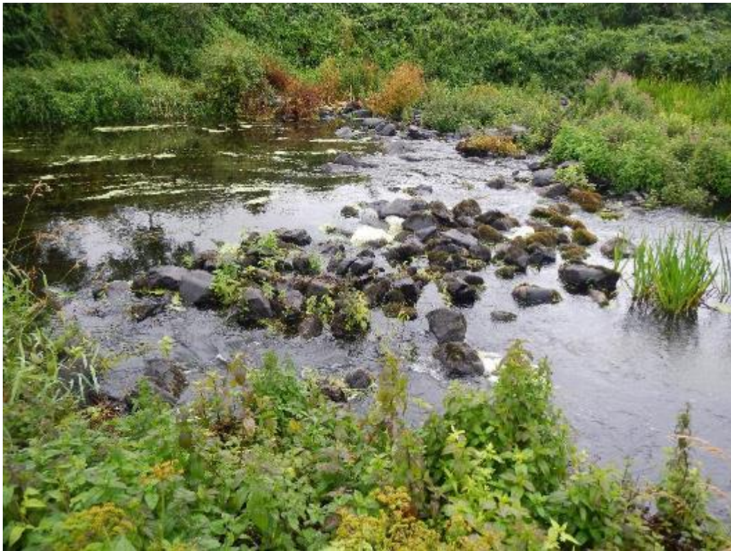
Photo 31. A more formal weir backs up flow and creates similar but greater issues as those found u/s (54.020598, -6.60211). Removing stones from the RB side would accentuate the existing left-hand bend and help consolidate flow and habitat alongside the island downstream. Otter spraint were observed at this point.
