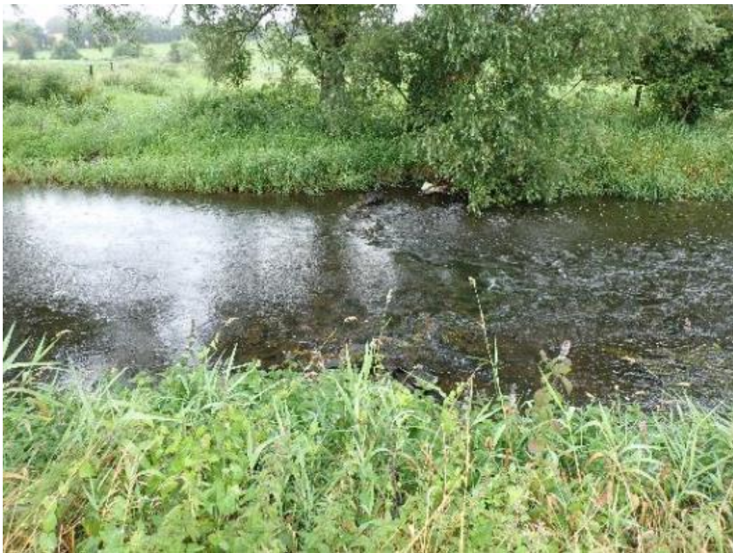
Photo 95. An old stone weir with the centre blown out: a much better outcome for the river. In such scenarios, it should be ensured that the foundations of the weir are also dislodged/removed to allow bed scour and depth creation.
