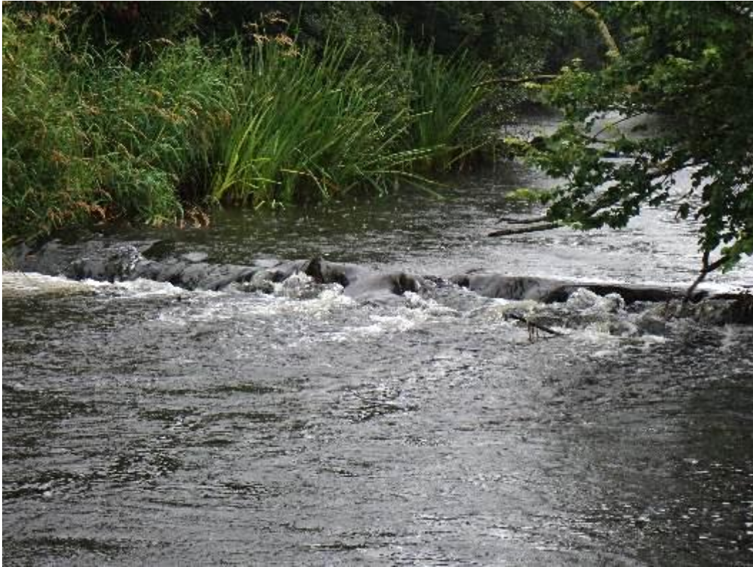
Photo 104. Yet another low stone weir is present on this reach (53.957936, -6.467749). Creating a 2m wide notch to be level is recommended.
