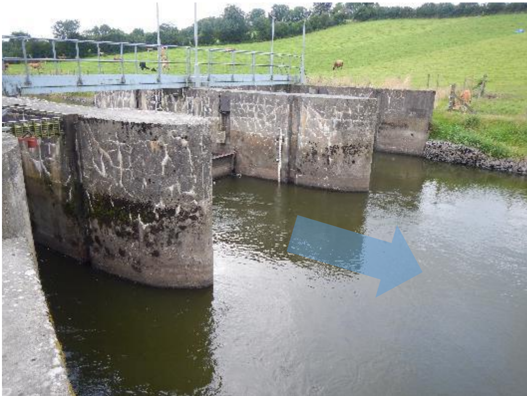
Photo 113. Looking at the d/s side of the structure: it appears some flow is also passing under the weir. This may provide some potential for fish passage, at certain times, but undershot structures are notoriously poor at facilitating d/s fish passage. Note the high turbidity of the water. Much of this is suspected to be algal/diatom growth, potentially indicating the enrichment/eutrophication recognised in the river system.
