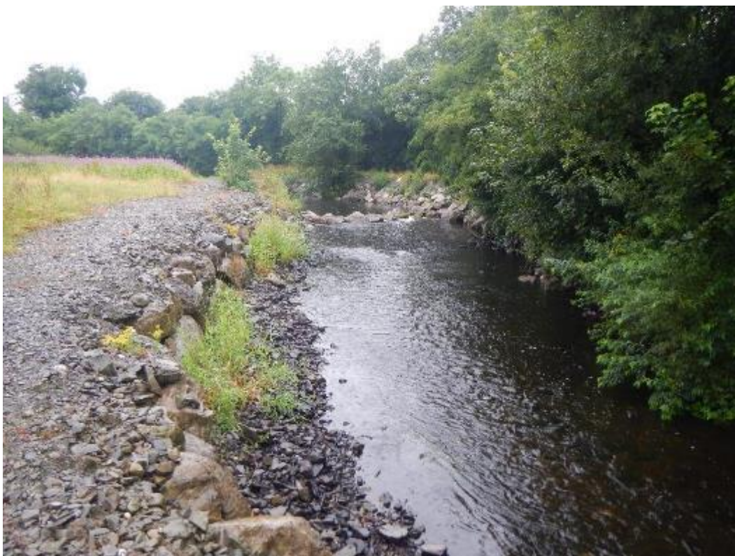
Photo 42. Spot checks were then undertaken around Inniskeen to look at some inappropriate in-channel work where weirs have been installed (54.004066, -6.582740). Dredging has also destabilised the bed and banks, leading to yet more bank work. It is not known what the purpose of the work was but it has certainly degraded the in-channel habitat for fish and interrupts vital sediment transport.
