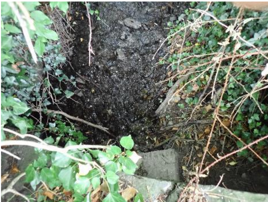
Photo 133. 53.978724, -6.517539 is the point at which the Carrickrobin disappears from view into a >100m-long culvert. This is likely to be a behavioural barrier to fish on spawning migrations, even if the culvert is not also a physical barrier to migration.
