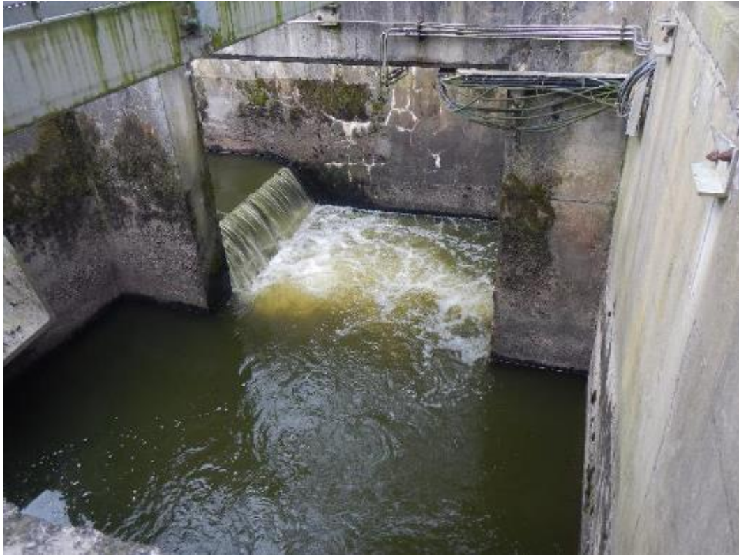
Photo 112. The air behind the over-spilling water prevents fish from swimming up through in the water column, requiring a well-timed leap to ascend the structure. The heavily aerated water immediately d/s also reduces the amount of force fish can create within the water to make the jump (i.e. the high content of air bubbles means there is less resistance for the fish to drive forward from).
