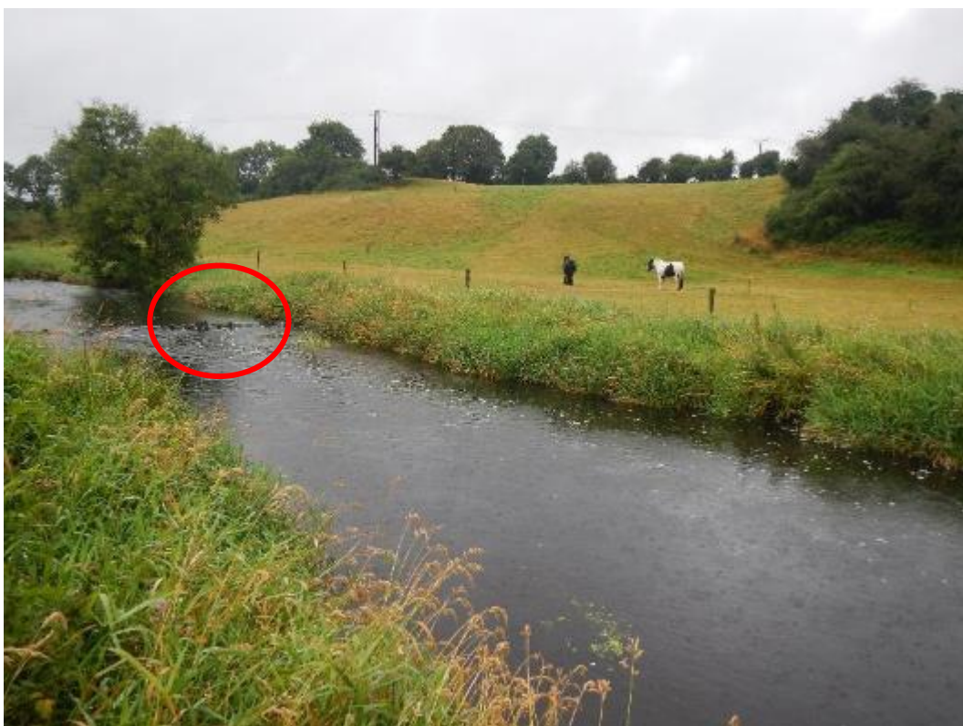
Photo 24. Small weirs in the river inhibit its natural flow pathways and trap bed material upstream (54.027212, -6.612428). Removing 1-2 metres of the weir right down to bed level at the LB side (red circle) would encourage flow in that area to create and maintain depth through scour. Where required, partial width deflectors are always preferable to full-width weirs. However, the lack of depth the weirs are intended to address would be better tackled through restoration of a more varied and sinuous channel.
