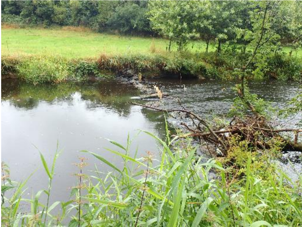
Photo 72. One of several low stone weirs in the Castlering to Knockbridge reach. Notching out a 2m wide gap to bed level would reinstate sediment transport and create an attractive flume for fish holding. Ideally, the gap should be on the side of the river where the flow velocities are potentially the fastest (outside of any sweeping bend).
