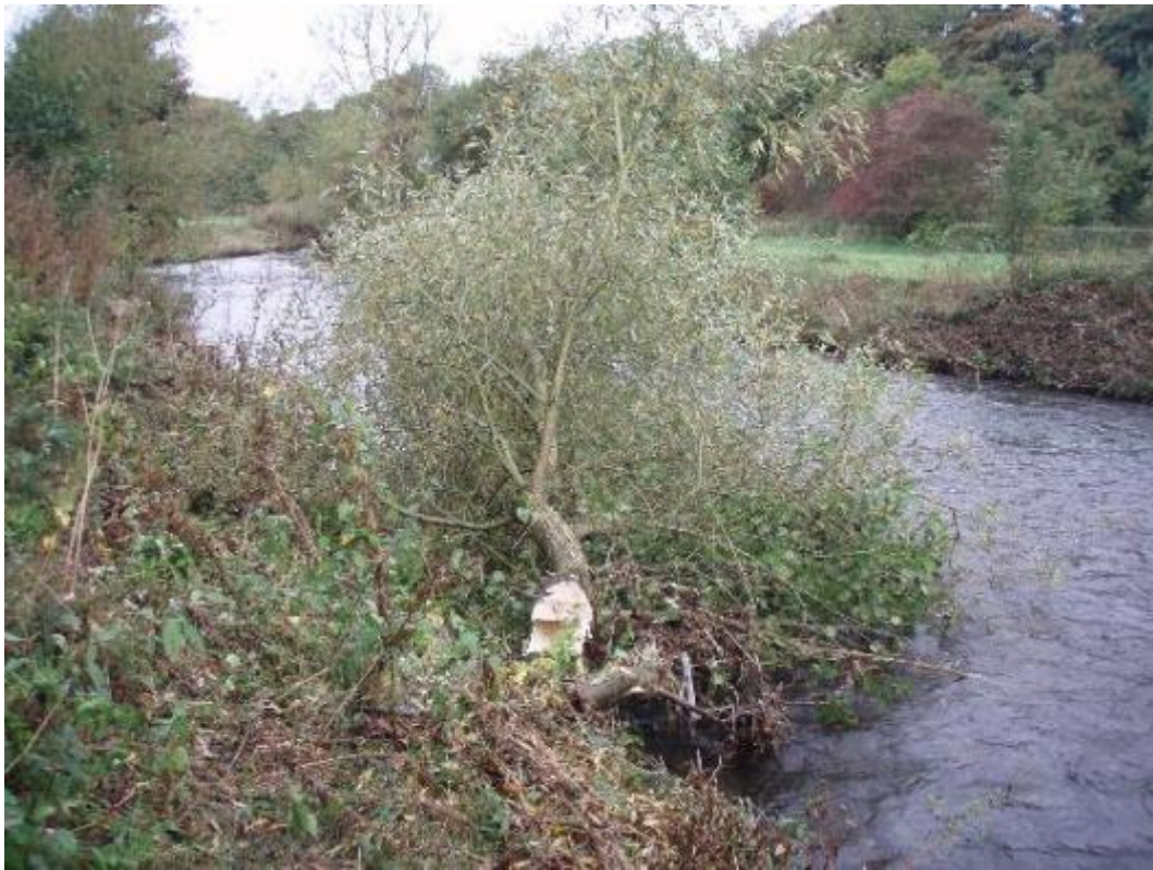
Photo 141. Example of a live willow hinged into the channel which will promote diverse changes in the bed shape of the river and provide cover for fish.
