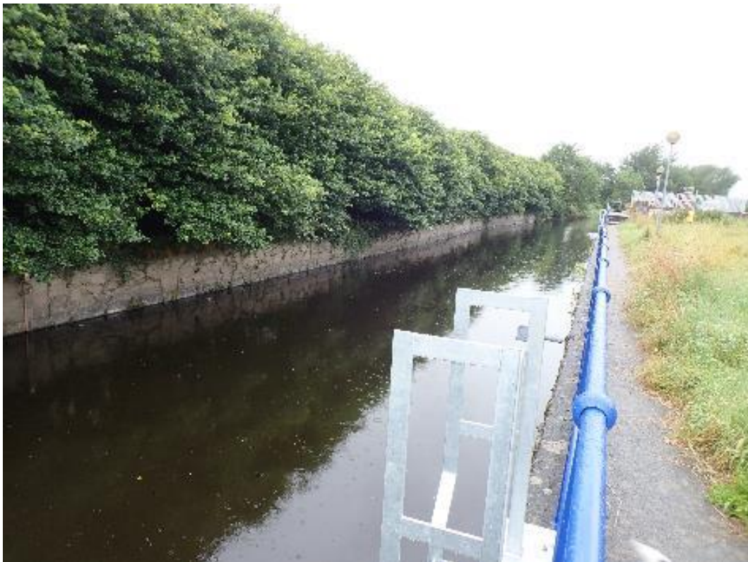
Photo 107. The long concrete channel constructed at the downstream end of the abstraction appears set up for flow gauging. It would be worthwhile ascertaining whether the data are available to the club. Dialogue with the regulators and water company might also identify if the long section of sterile channel could be improved via box planters to provide shade and cover without interfering with the laminar flows within the gauging box.
