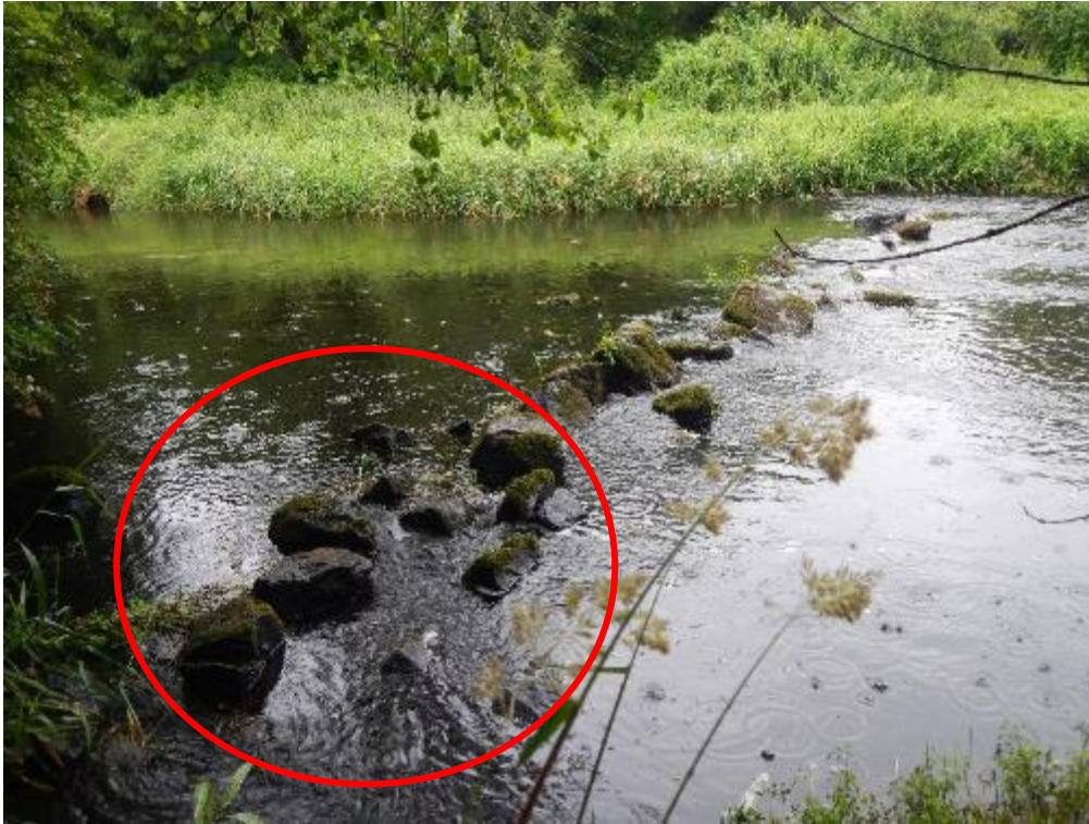
Photo 25. A weir a short distance d/s creates a similar issue (54.025323, -6.609878). Here, removing 1-2 metres of the weir down to bed level at the RB side (red circle) would encourage flow along the RB. When removing part of a weir (or installing deflectors), it is important to maintain the movement of the flow from one bank side to the other, to avoid effectively straightening the flow. It is therefore also important to consider which side of the channel the flow would naturally approach from u/s when choosing which side to notch.
