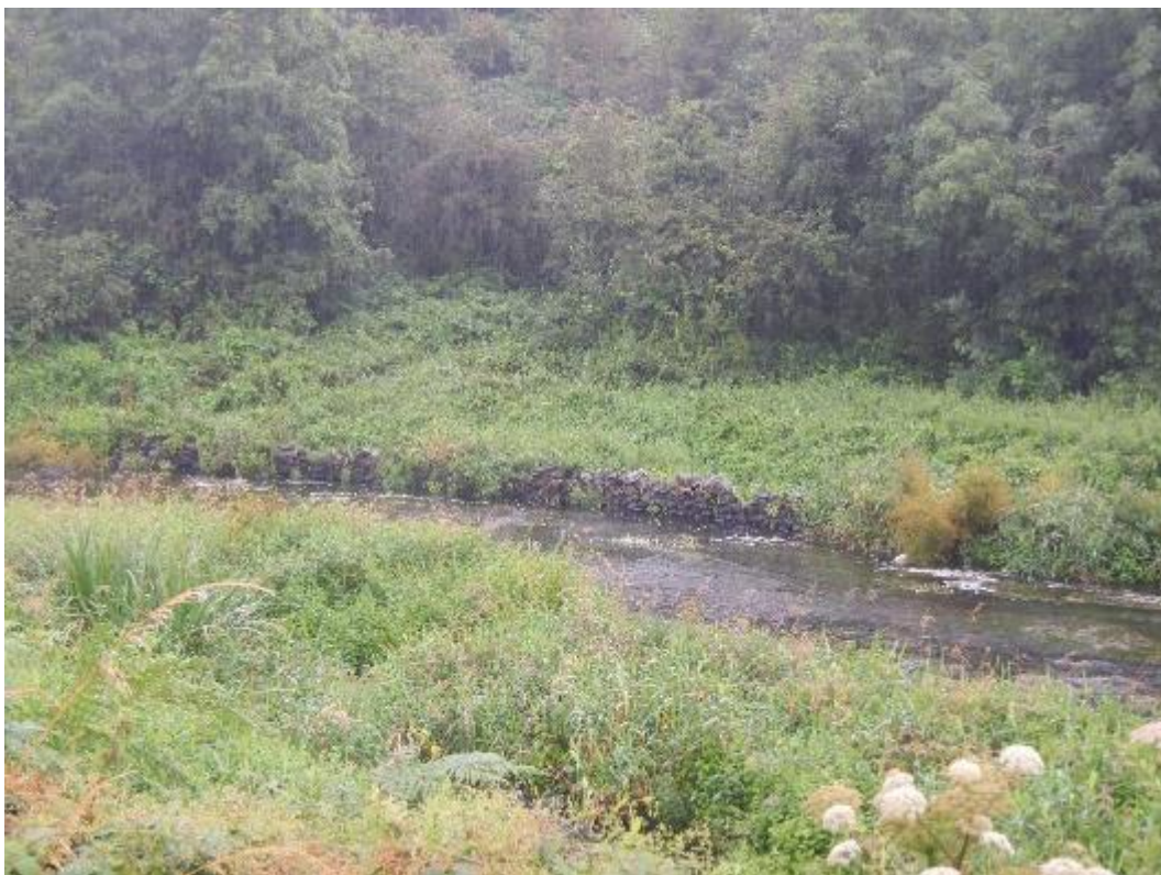
Photo 28. Armouring of the LB could be removed to allow natural, lateral movement of the channel into the rough ground on the outside of the bend (54.024075, -6.606928).
