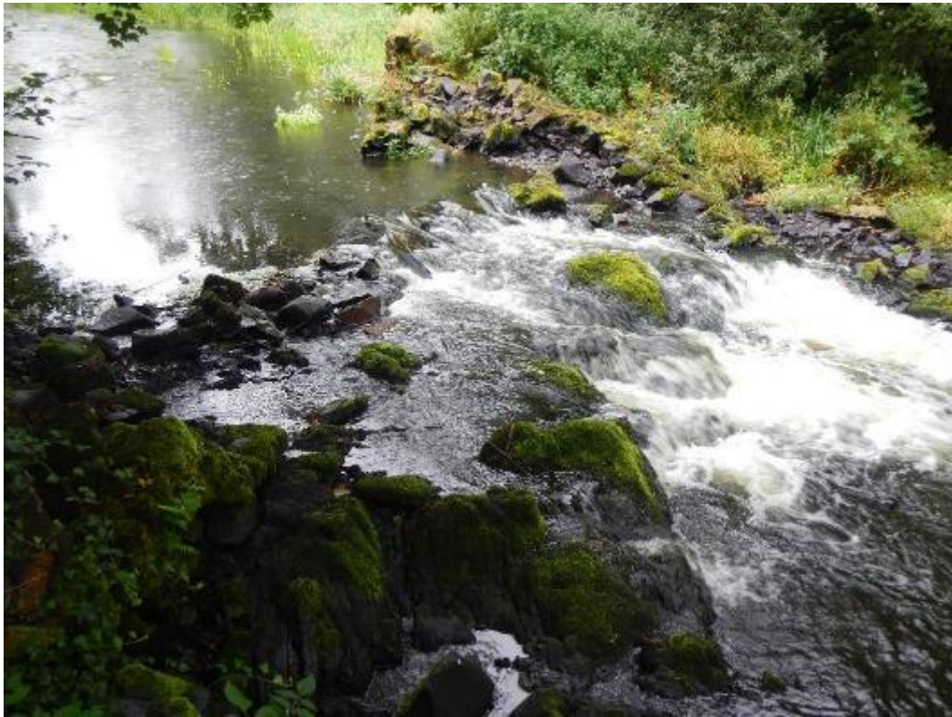
Photo 1. A spot-check was undertaken on the upper River Fane, visiting a collapsed weir (54.059055, -6.647277). The underlying bedrock creates a small natural obstruction but passability is made worse by the weir, and subsequent attempts to rebuild it. Ideally, the manmade part of this structure should be removed or allowed to fully disintegrate.
