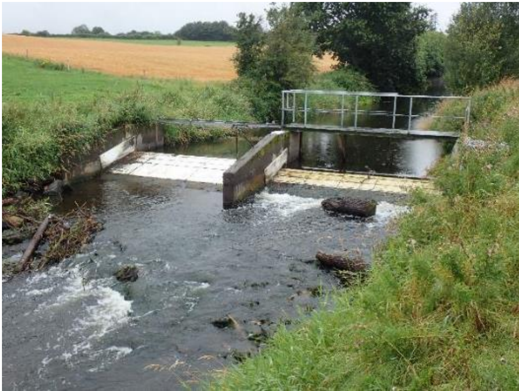
Photo 109. The crump weir/fish counter located a short distance downstream of the abstraction point (53.9536604, -6.4580669) raises a number of questions:
