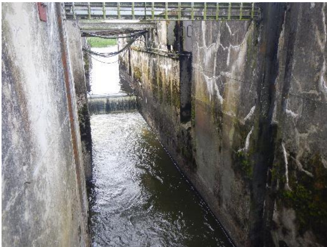
Photo 111. The dam just d/s of Lough Muckno (54.099668, -6.67637) regulates flow in the Clarebane River. The overspill of the weir and narrow approach create an obstruction to fish movement u/s and the abrupt lift and flow constriction almost certainly inhibits d/s fish migration, particularly for smolts whose run-timing can be critical for successful seaward migration. Again, the delays also increase predation and disease risk.
