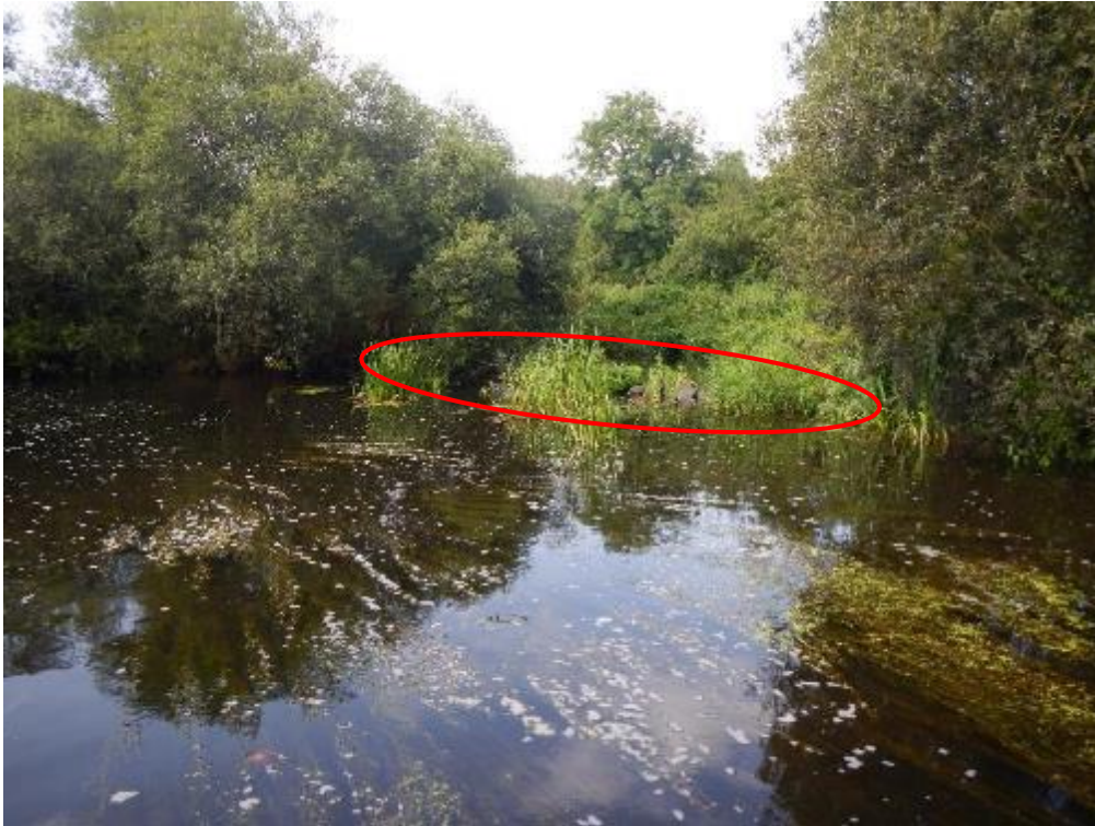
Photo 21. Rocks have been used to reduce the flow passing down the side channel (red ellipse). The pool at the d/s (foreground) would change if the predominant flow came down the side-channel, but the overall habitat diversity and quality would be increased.
