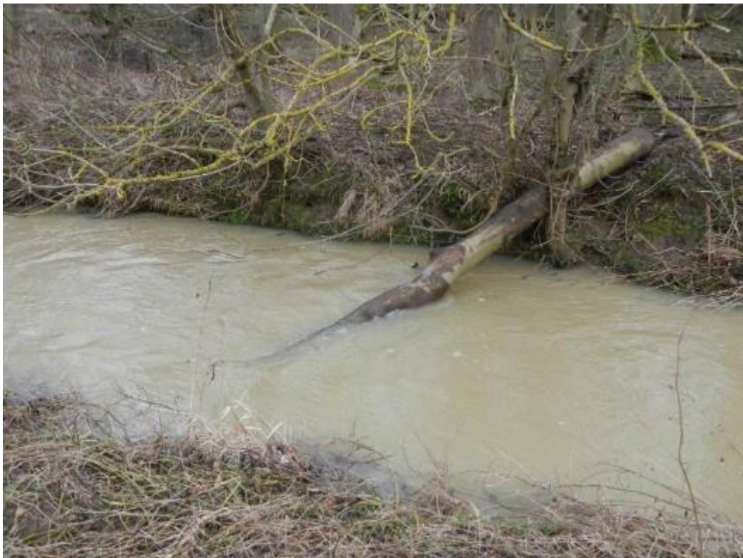
Photo 142. A lodged flow deflector – the technique can be used with a single trunk or branch (primarily to increase scour) or a multi-branched limb (to create greater flow dissipation and more in-channel structure). The elevated butt end (bank end) reduces the potential for detrimental bank scour (usually associated with d/s deflectors) as a through-flow is maintained along the bank.
