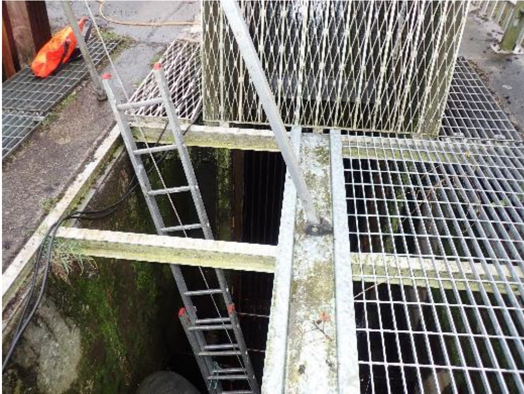
Photo 106. The chamber to the public water supply abstraction near the bottom of the beat (53.954030, -6.460303). The author was surprised to find that there were only trash screens and appeared to be no fish barriers or behavioural screens installed. It is highly likely that this intake will be entraining smolts and eels on migration. Dialogue is required to establish if screens are fitted and if not, lobby for urgent mitigation.
